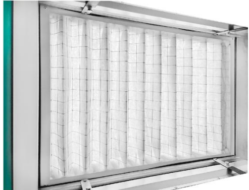
Picture 21 (b) General view of a cassette filter in a section
